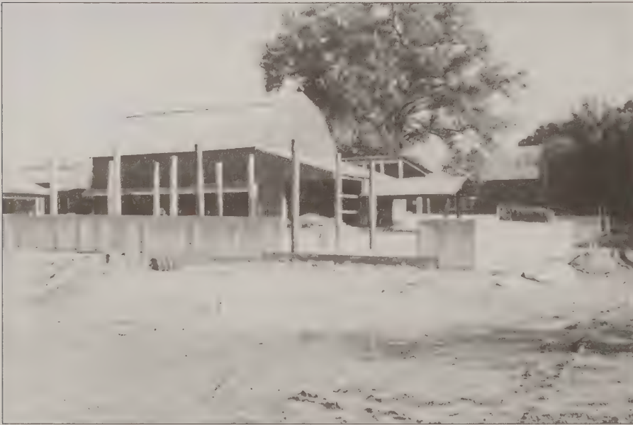
Construction of Animal Waste Storage Structure
